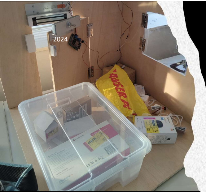
central unit box
