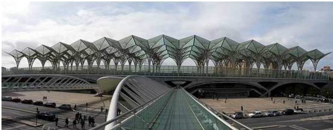
Figure 6.201 – Overview of Gare do Oriente Intermodal Terminal
