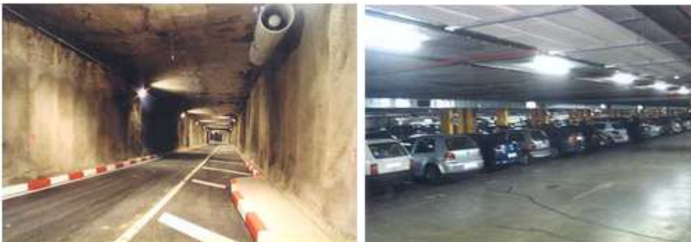
Figure 6.44 Tunnel and car parking at the Interchange.
