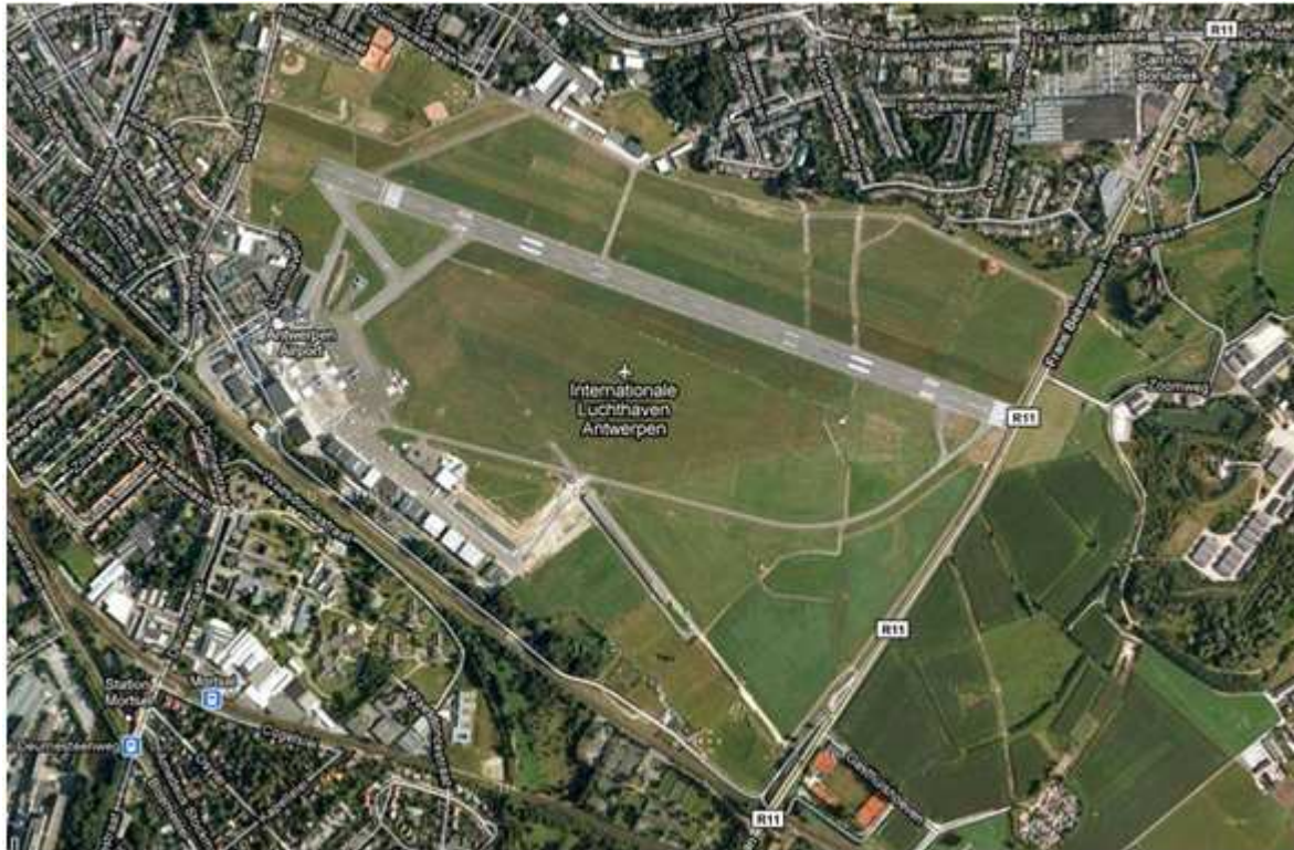
Figure 6.288 Aerial photo of Antwerp Airport Source: Google Maps
