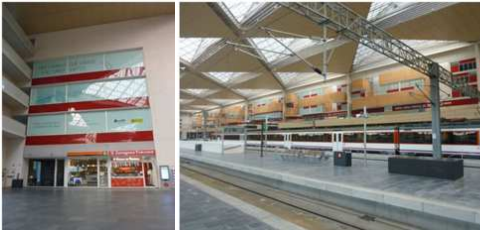
Figure 6.113 Zaragoza Interchange: lobby for arrivals
