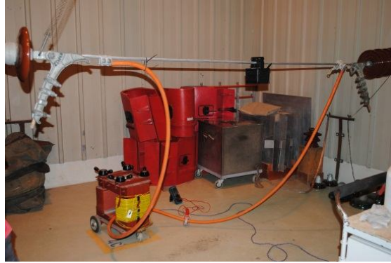
Fig. 4. High Voltage Tests
