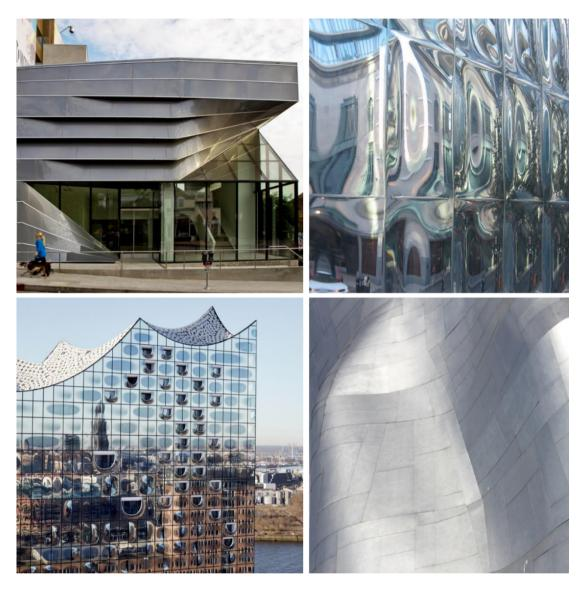
Figure 6.5. Formative manufacturing examples (from left to right): Prism Gallery by P-A-T-T-E-R-N-S, 2010 (©P-A-T-T-E-R-N-S); Holt Renfrew flagship store in Vancouver by Janson Goldstein Architects, 2008 (©Marc Simmons / Front Inc); Elbphilharmonie Hamburg by Herzog & de Meuron, 2017 (©Maxim Schulz); Experience Music Project by Frank Gehry, 2000 (©David via Blogger "Doodles Designs and Daydreams").
