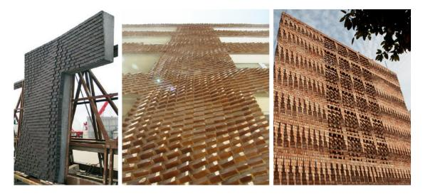
Figure 6.23. From left to right: a brick panel of the 290 Mulberry Street building facade produced in a factory and then transported to the project's site to be assembled [355]; DIY For Architects brick facade (©Sstudiomm); South Asian Human Rights Documentation Centre (©AnagramArchitects).
