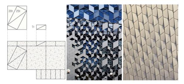
Figure 6.22. From left to right: the triangular tilling rule of the Federation Square facade (edited from [47]); the diamond-shaped facade of Lane 189 (©Eric Jap); MAAT facade tiles (©HUFTON+CROW / AL\_A).
