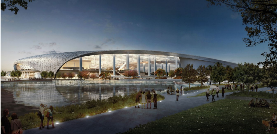
Figure 19. The porous canopy of SoFi stadium composed of approximately 35 000 anodized aluminium panels with different perforation patterns (from [63]).
